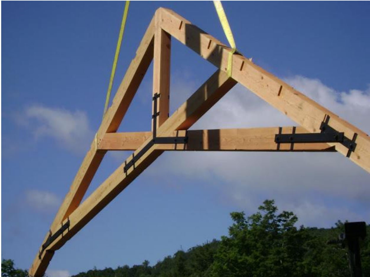
Pinned straps on scissor truss
