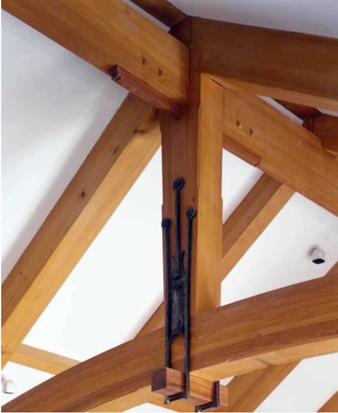
Curved glulam bottom chord for Norm Abram's great room
