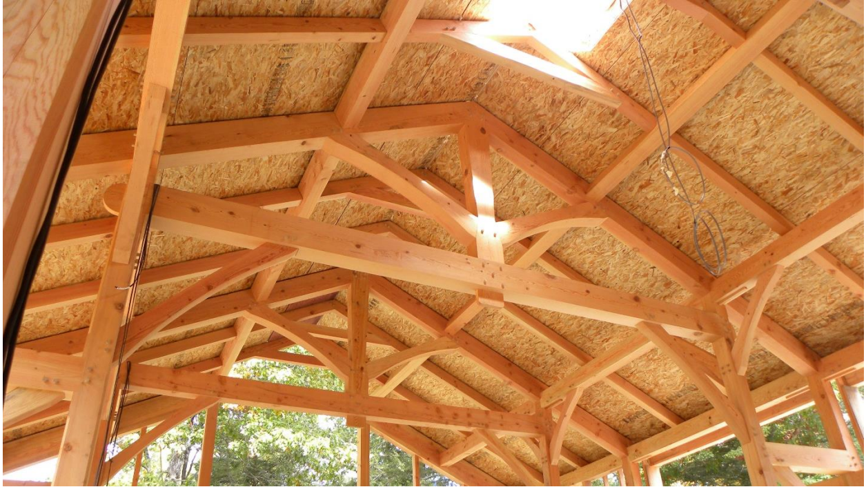
Howe truss with a dropped bottom chord
