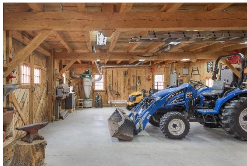
Example of a queen-post truss supporting the second-floor structure of a barn to provide a column free space below. Purlins supporting roof rafters rest on the queen-posts.
