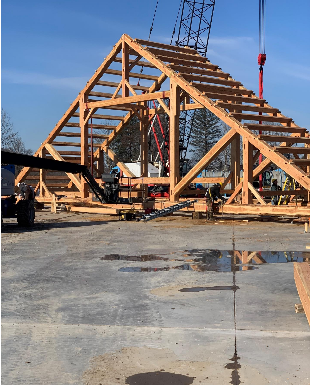
80-foot span queen-post trusses
