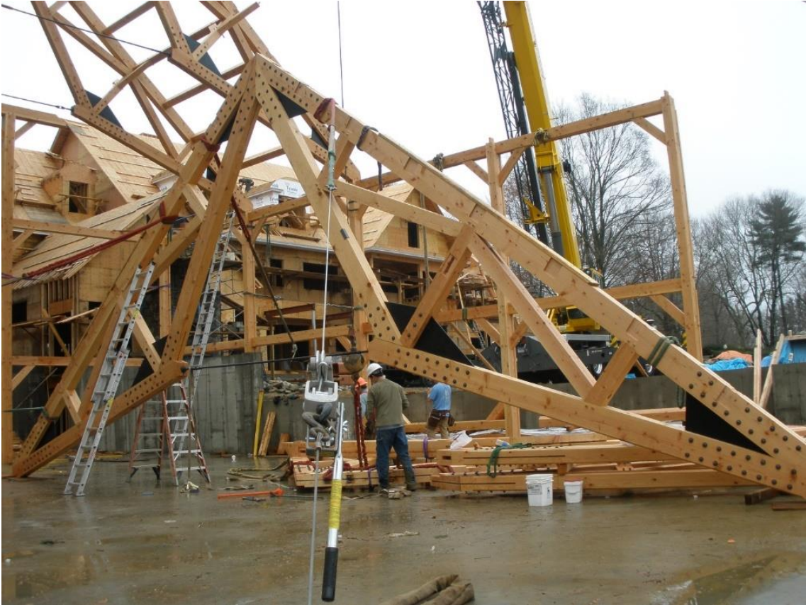
Compound Fink truss made up of two smaller trusses joined in the field.
