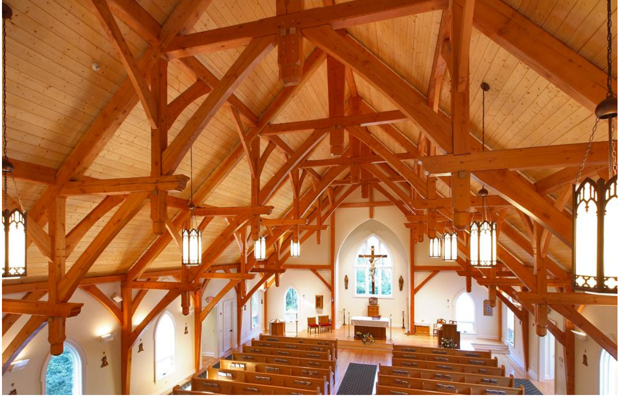
Example of a contemporary hammer-beam structure. Saint Patrick Church, Redding, Connecticut.
