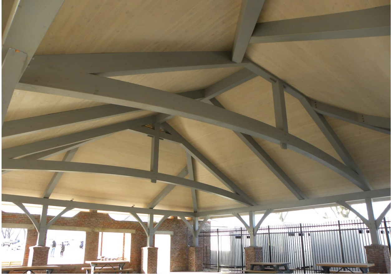
Glulam trusses with curved bottom chords
