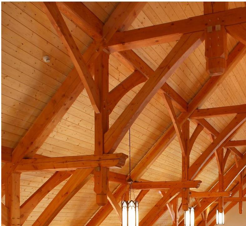
Hammer-beam trusses braced to roof purlins
