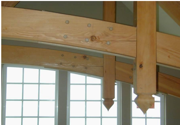
Seasoning checks indicate the grain orientation.
