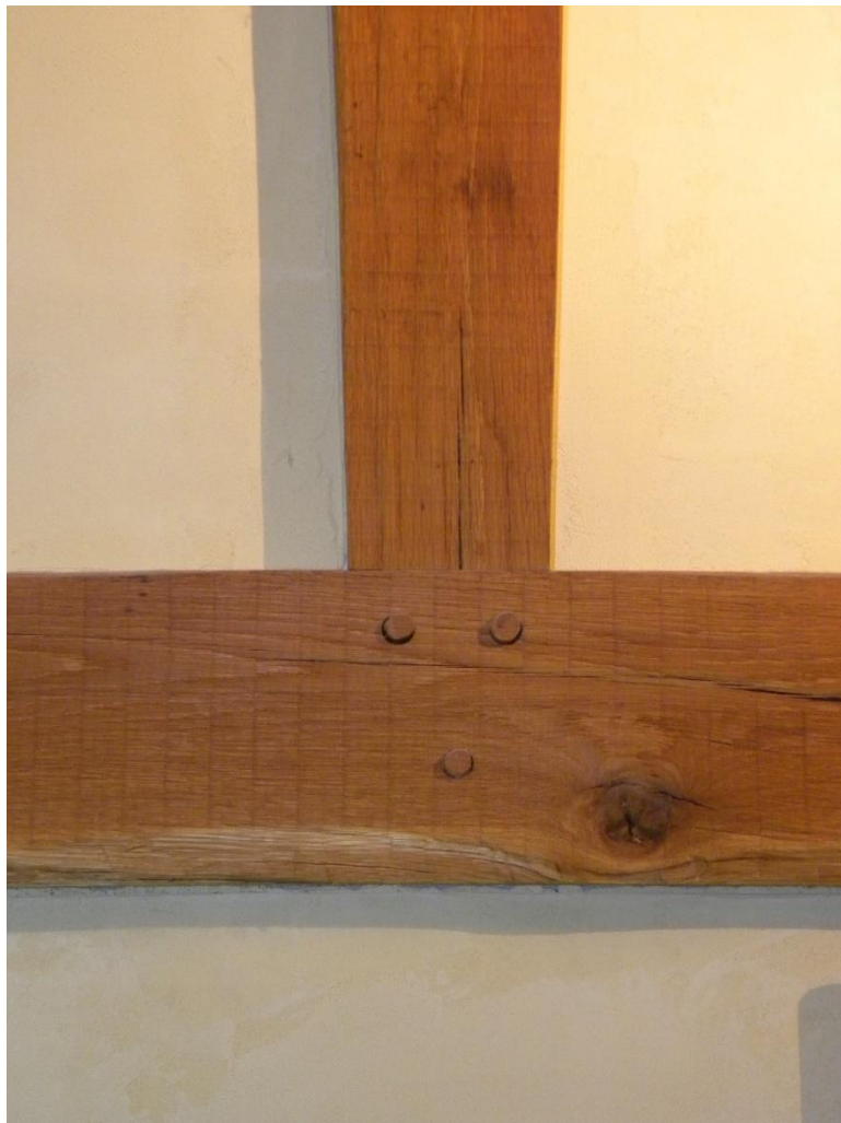
Pegged mortise and tenon king-post connection to a bottom chord
