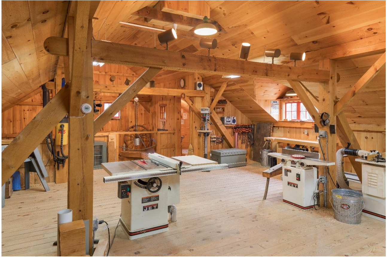
Example of a queen-post truss supporting the second-floor structure of a barn to provide a column free space below. Purlins supporting roof rafters rest on the queen-posts.
