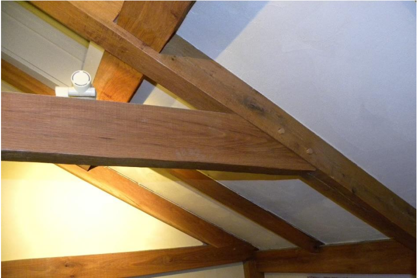
Raised bottom chord aka "the rafter buster"
